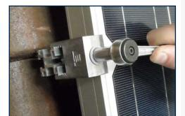
6. Mounting the first panel on the mounting rails
